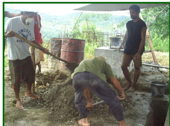
Immediately after the welded foundation was delivered, the Concrete Team started mixing the concrete and filled up the hole. Two men kept the concrete moving by stirring it with long sticks. This is to release air and upgrade the concrete's quality. As they reached the instructed level, Bas monitored placing the iron foundation. Then the workers added concrete and worked until way after dark, as all concrete had to dry in one massive block. It takes at least two days to dry.
