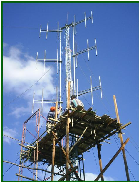
Step by step, the eight elements and the antenna cable (through splitters attached with tie-raps) were attached to the new construction. After every two elements, the tower was raised to the next level. The antenna elements were attached in an angle and direction that allows the signal to reach as many villages within Viqueque District as possible (away from the sea). The tower was growing higher bit by bit, and became visible for the people down at the market.
